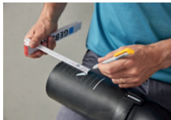
The Geberit Silent-Pro BottomTurn bend can be easily adapted to the ceiling thickness.
