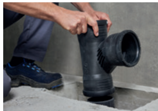
A drainage system with Geberit Silent-Pro SuperTube is plugged together.
